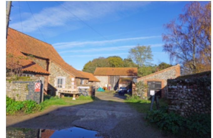
Yard surrounded by barns
