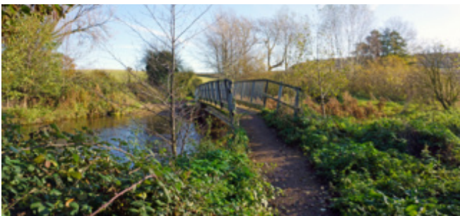
The bridge over the ford
