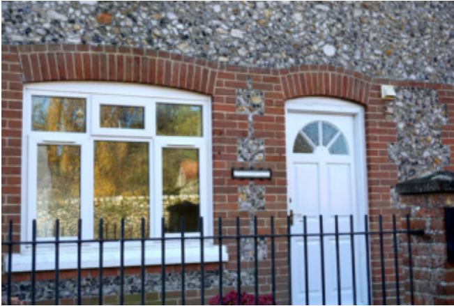
uPVC window and modern replacement door
